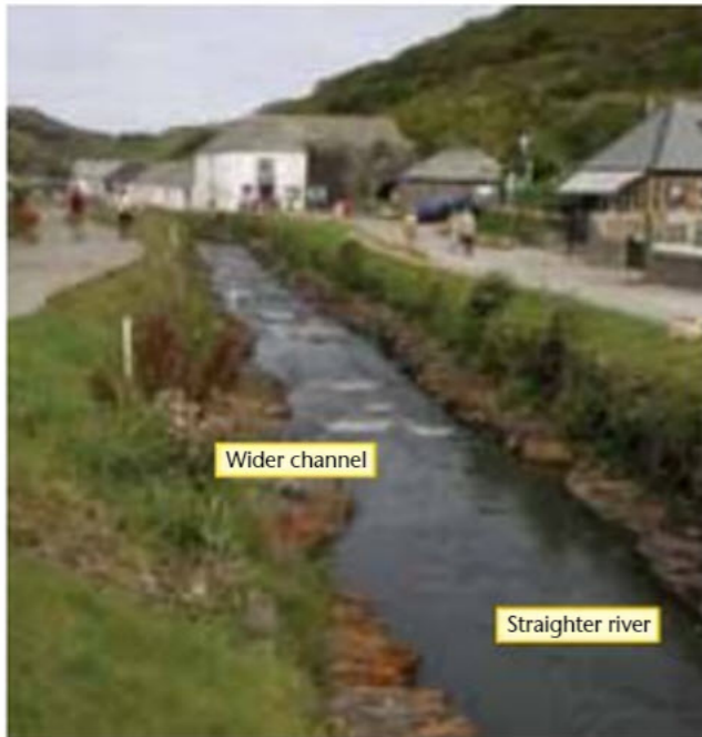
▲ Figure 17 The section of river between the main bridge and the harbour has been lowered by 75 cm. The river has also been widened.
