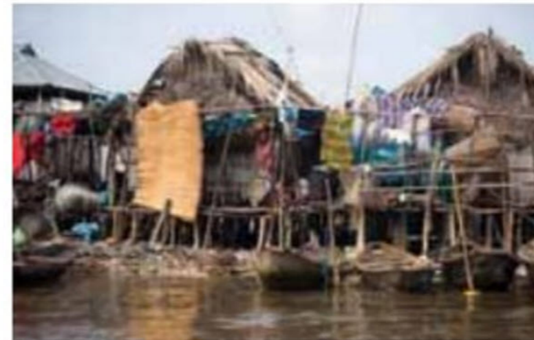
▲ Figure 28 Poor neighbourhoods in Cotonou, Benin are built on stilts along the waterfront.
