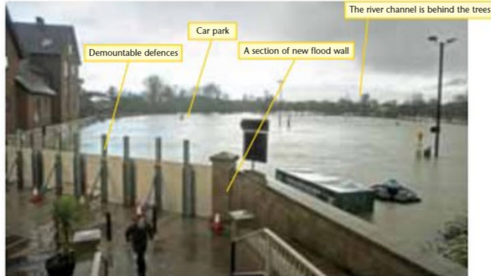
▲ Figure 30 A total length of 700 m of flood embankments and walls has been built where the river enters the town to prevent floods in Shrewsbury. A further 155 m of river bank is protected using demountable defences.
