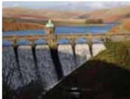
▲ Figure 2 The Penyarreg reservoir and the Craig Goch dam in the Elan Valley.
