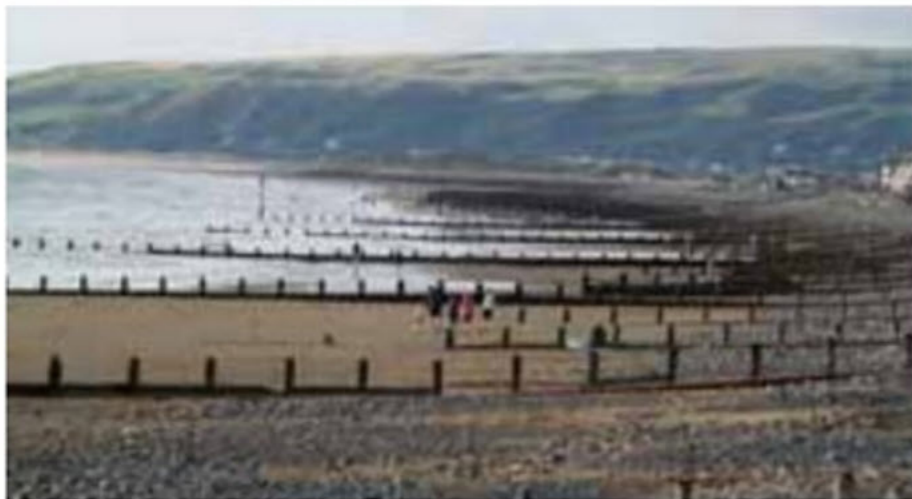
◀ Figure 10 Wooden groynes on Borth beach in 2008.
