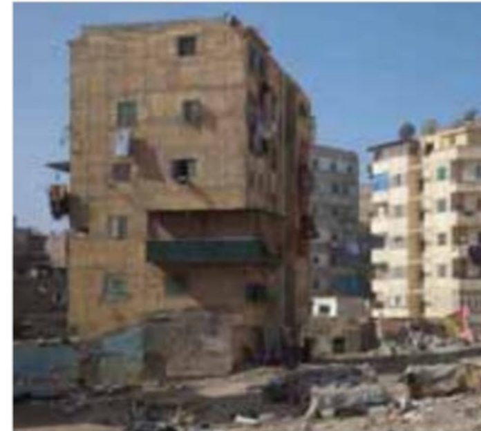
▲ Figure 25 Illegally built flats in Alexandria, Egypt.
